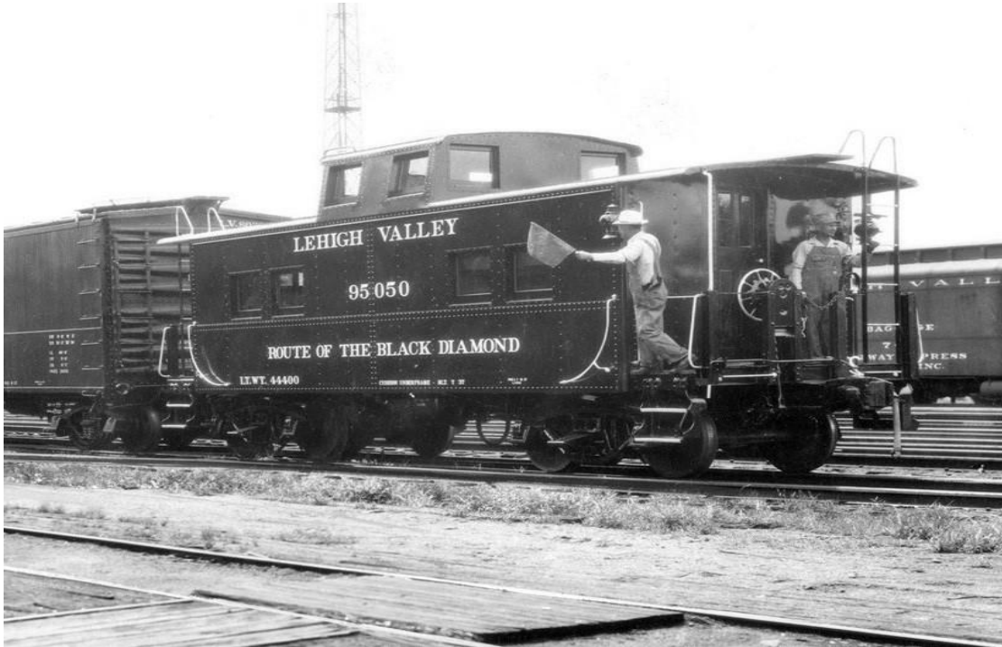
LV 95050 at Unknown Location in 1937 (LVRR Photograph, Railroad Museum of Pennsylvania Collection)
